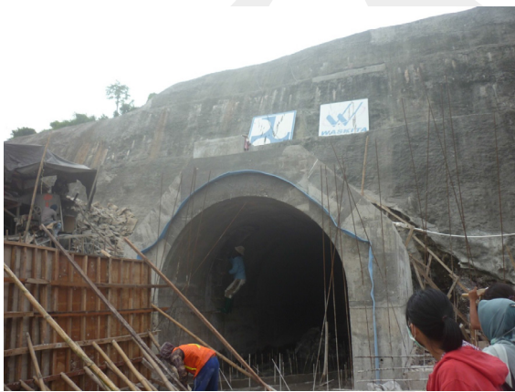
Figure 2. Pandan Duri tunnel under construction.
