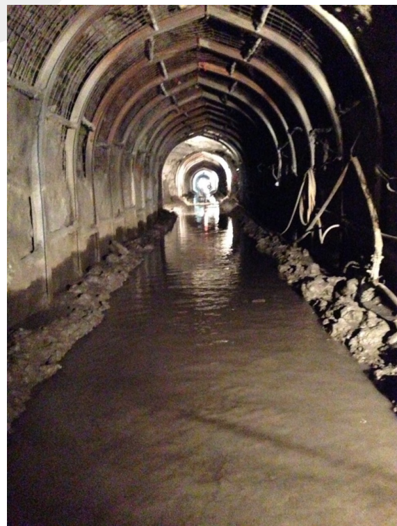
Figure 3. Mila tunnel under construction.
