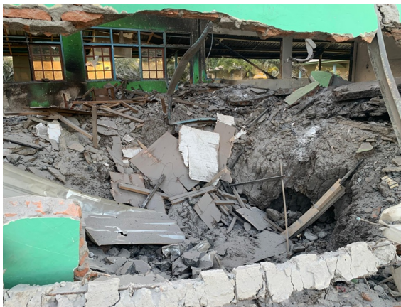
Figure 5. The impact of blast material of Lewotobi Laki-laki eruption on 3 rd November 2024, at 23:57 Central Indonesia Time on school building.
