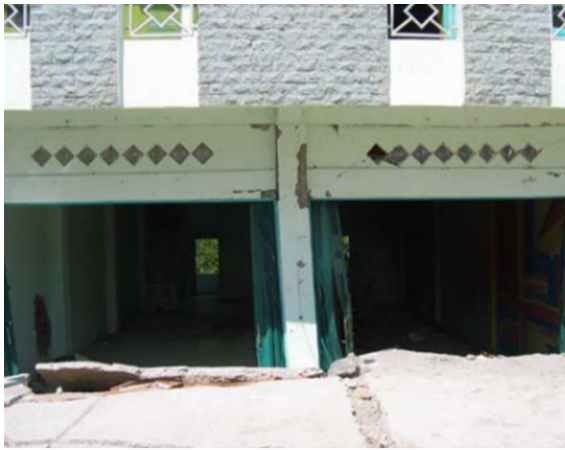
Figure 4. Evidence of liquefaction events in Tanah Patah (after Hausler and Anderson, 2007).
