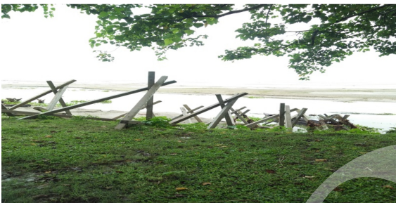
Figure 13. Photograph of installation of porcupine method in Minalpur Village.
