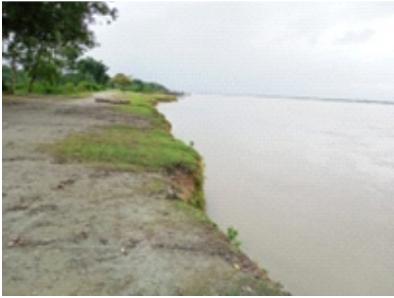
Figure 6. Photograph of bank erosion (Rohmorria).
