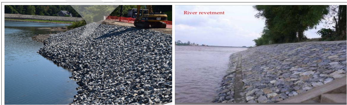
Figure 11. Photographs of riprap or rock fills/river revetment (Poa St. James. Erosion Control and Pond Bank Stabilization Methods).
