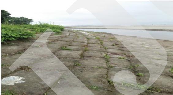
Figure 9. Photograph of Minalpur Village using geotextiles technique. Anti-erosion works along with the left bank of Jiabharali River, Assam Manish Gupta, Suresh Maurya, and Chitra River, Central Soil and Materials Research Station (CSMRS), New Delhi- 110016.
