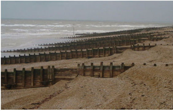
Figure 12. Photographs of groyne structure.
